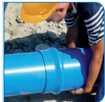
Firmly push the free end into the other pipe. Introduce until the end marked is no longer seen.
