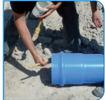
Apply lubricant on the chamfer of the spigot end and in the rubber ring joint.
